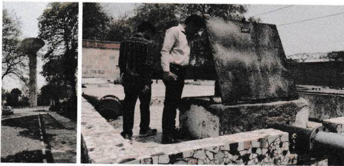
Underground and overhead tank in campus for water supply
