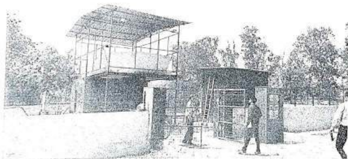
Waste to Energy Plant in DTU campus near water pond area
